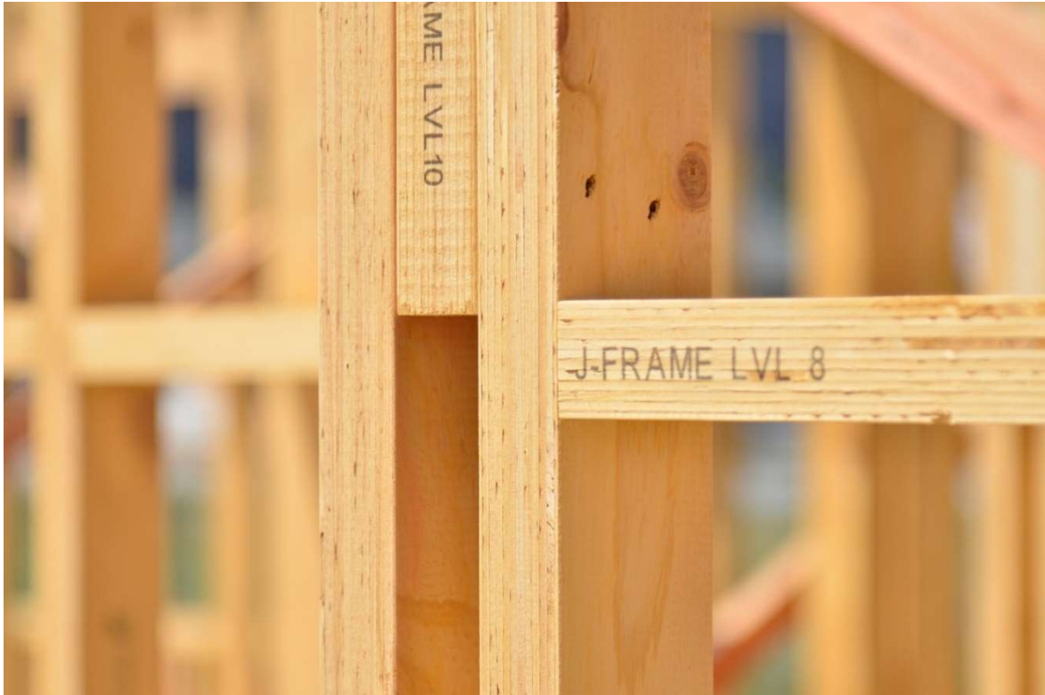
Figure 6: Structural LVL product example. Adopted from Zealand [40].
