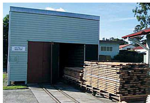
Stack ready for drying in a solar kiln. Weights still to be added.
