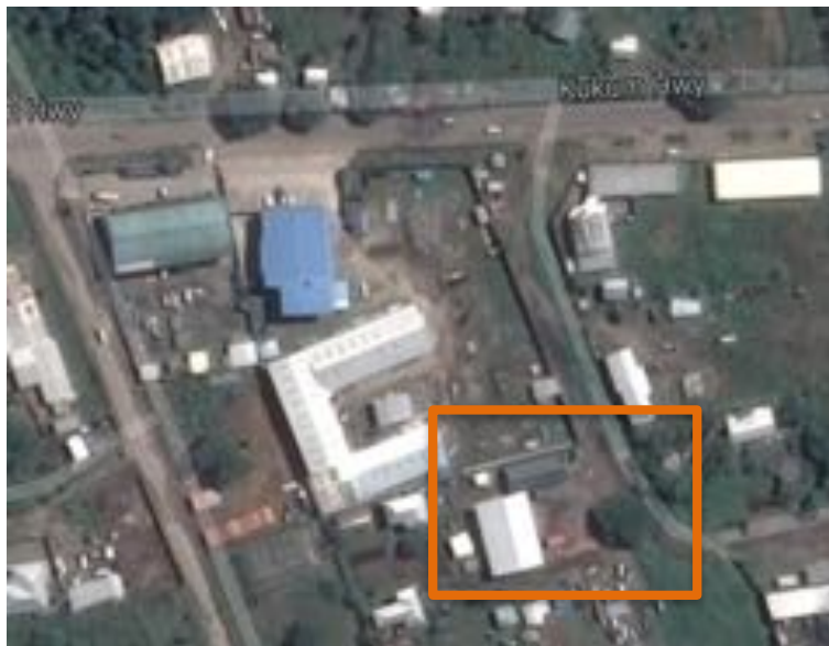
Figure 7: Aerial view of the VATA facility.
