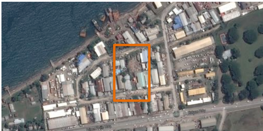
Figure 4: Aerial view of the Timol Timber facility.
