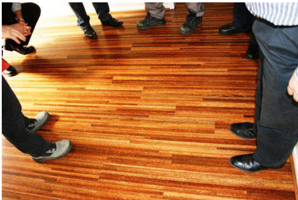
Image 1. Engineered flooring combining sawn coconut and plywood.
