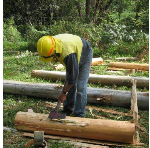
Figure 4.4 Removing bark from hardwood billets with the cutting face of the axe.
