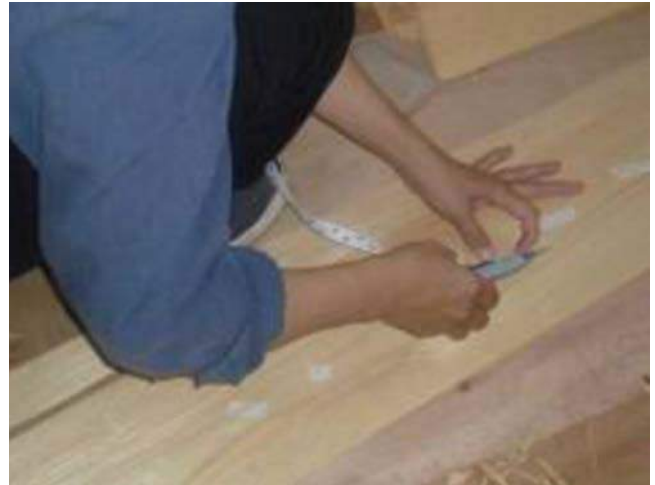
Figure 7.16 Veneer taping.
